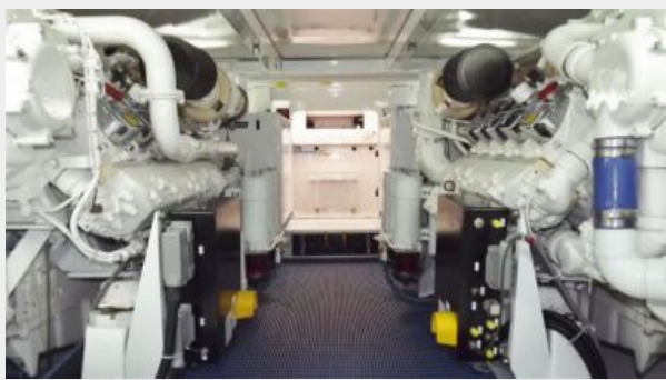
Engine Room Aft
