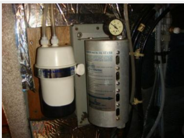
44' Tollycraft engine room starboard forward
