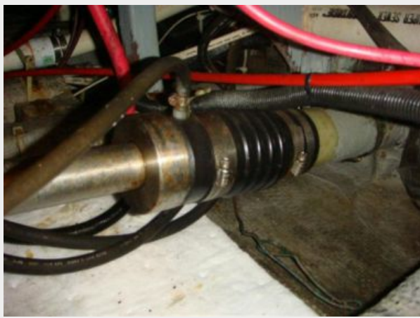
44' Tollycraft starboard shaft seal
