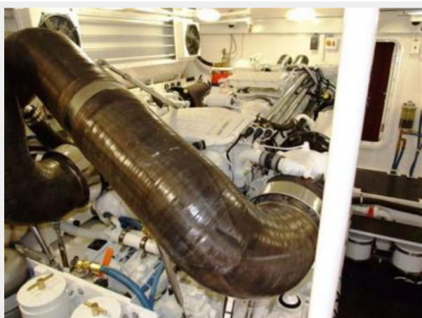
Engine Room Port
