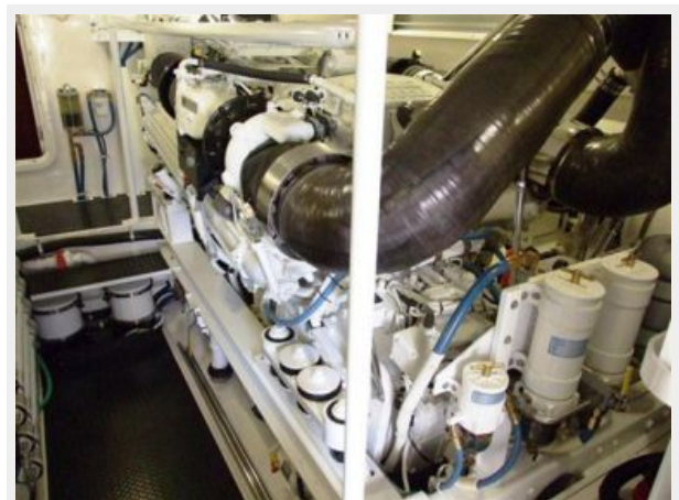
Engine Room Starboard
