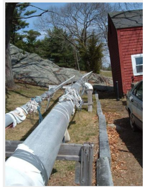
Mast w/radar mount
