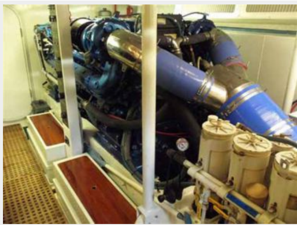
Starboard Engine Room
