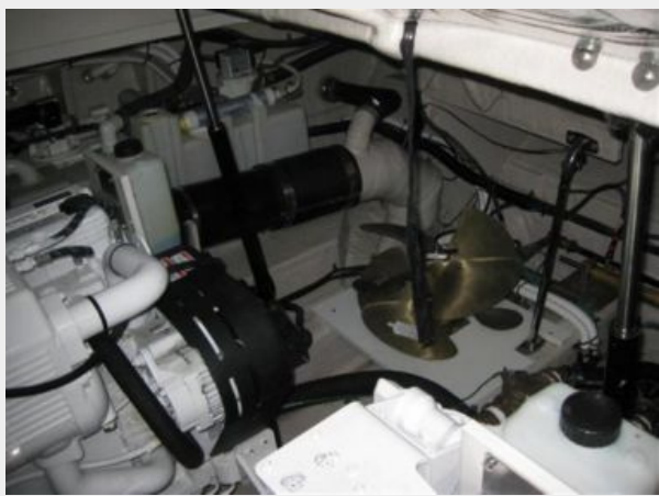
Engine Room w/ Spare Props
