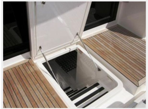
Engine Room Access
