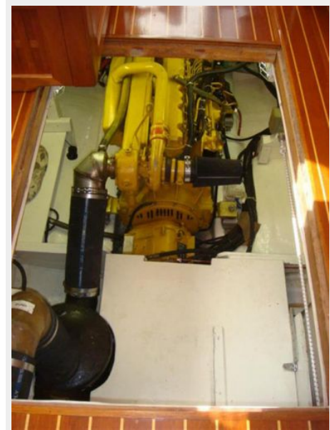
44' North Shore Trawler engine room
