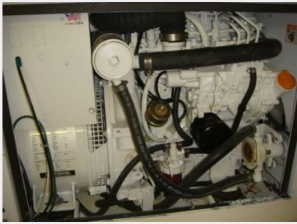
44' North Shore Trawler generator
