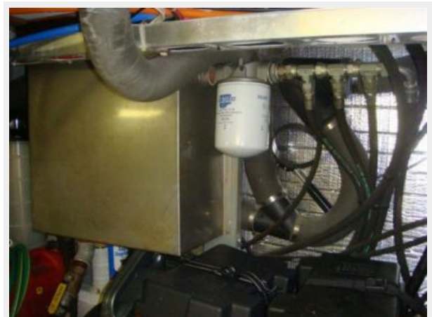
44' North Shore Trawler hydraulic system
