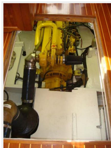
44' North Shore Trawler engine room
