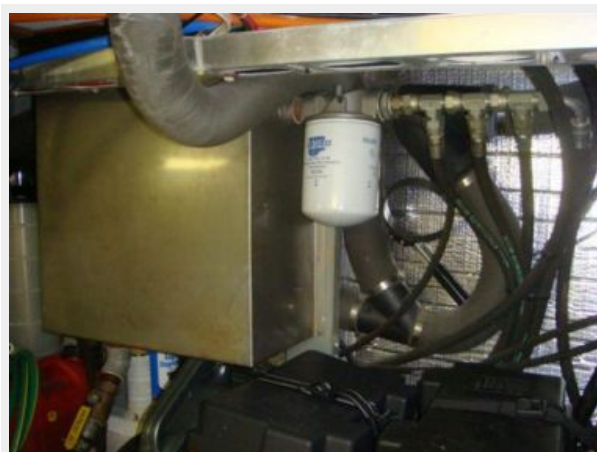
44' North Shore Trawler hydraulic system
