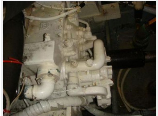
70' Hatteras Motoryacht starboard gearbox
