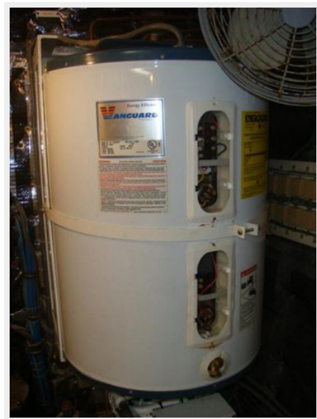
70' Hatteras Motoryacht port water heater
