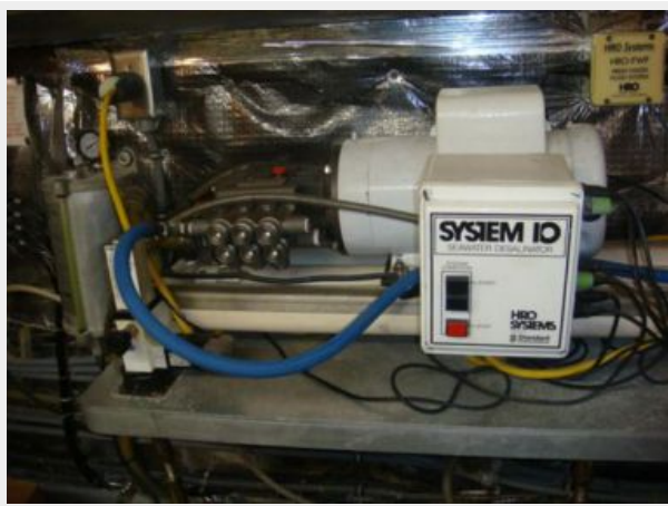
70' Hatteras Motoryacht watermaker
