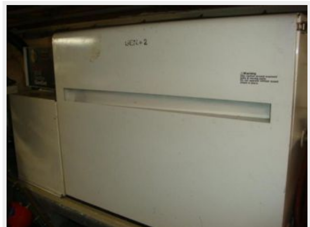
70' Hatteras Motoryacht generator2 soundbox
