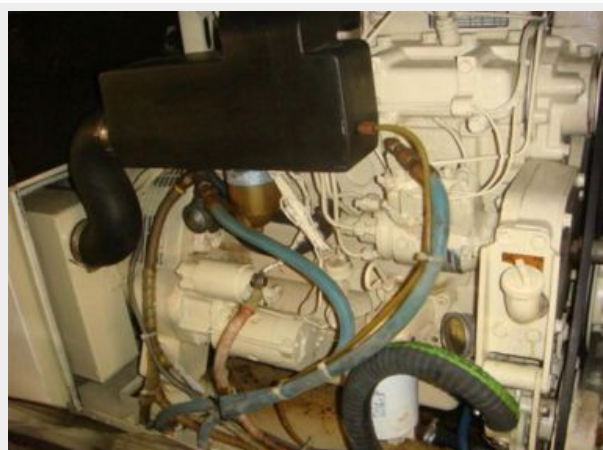
70' Hatteras Motoryacht generator2
