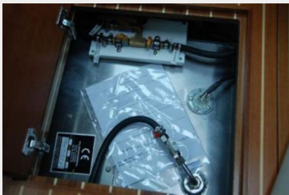
Extra Diesel Tanks
