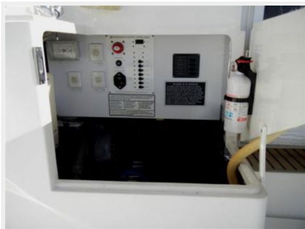
Engine room access
