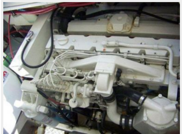
Engine and Mechanical Equipment 2
