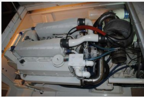
Starboard Top Engine
