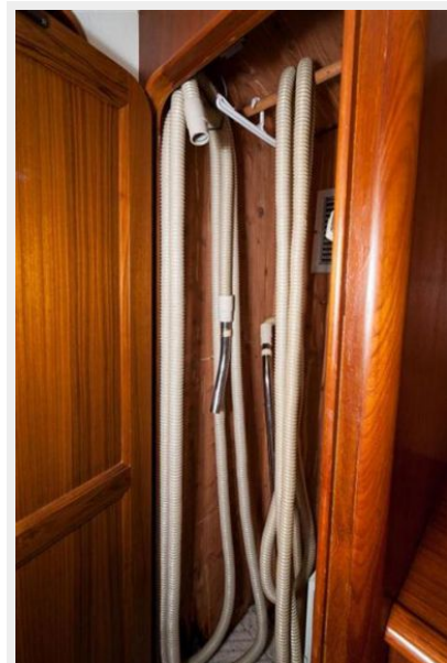
Central Vacuum System
