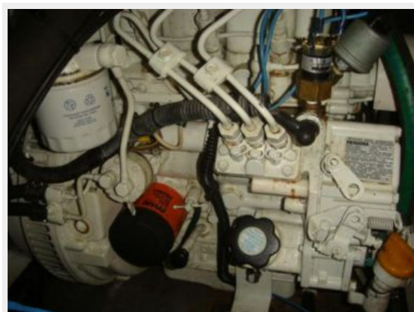
42' Hunter generator photo1
