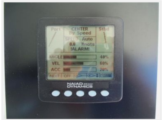
New Stabilizer Controls
