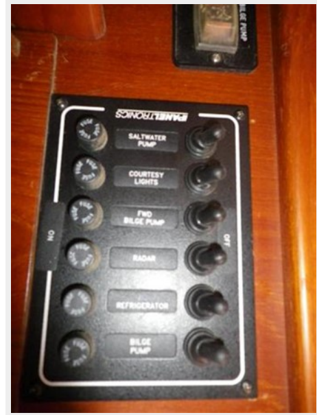
Bilge pump panel
