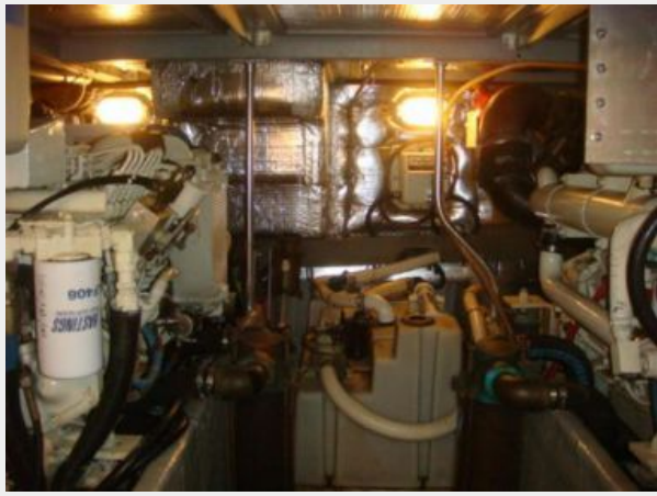
43' Mainship engine room
