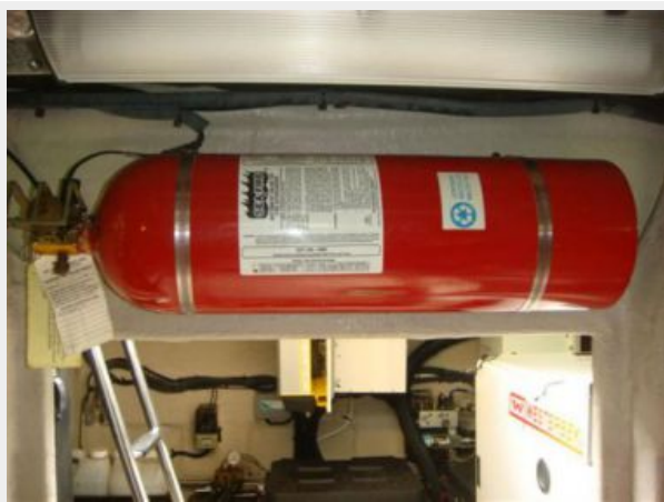
54' Sea Ray fire suppression system
