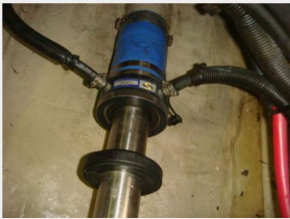
54' Sea Ray starboard shaft seal
