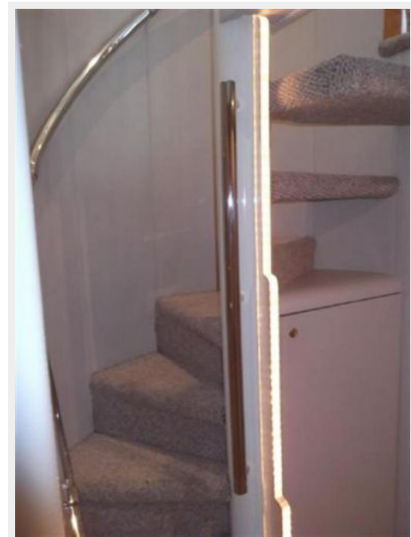
Central Vacuum System Under Spiral Staircase
