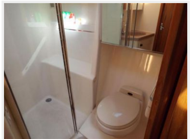
40' Tiara Vacu-flush head
