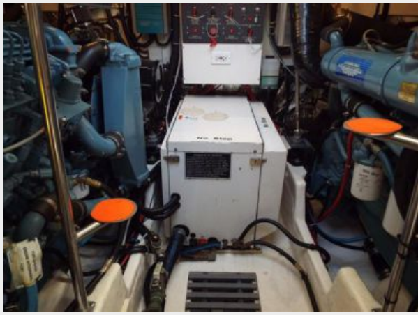
40' Tiara engine room forward
