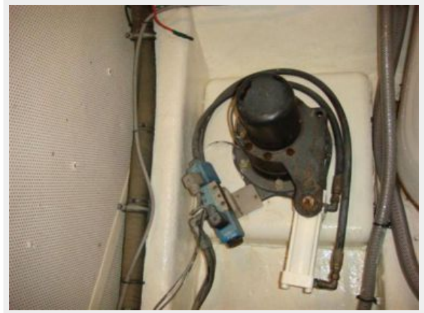
55' Ocean Alexander starboard stabilizer head
