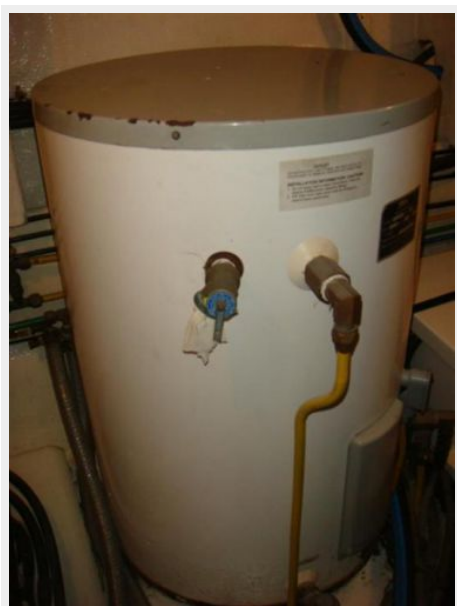
55' Ocean Alexander water heater
