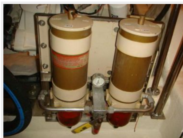
55' Ocean Alexander starboard Racor fuel filters
