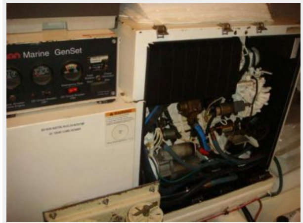
55' Ocean Alexander generator
