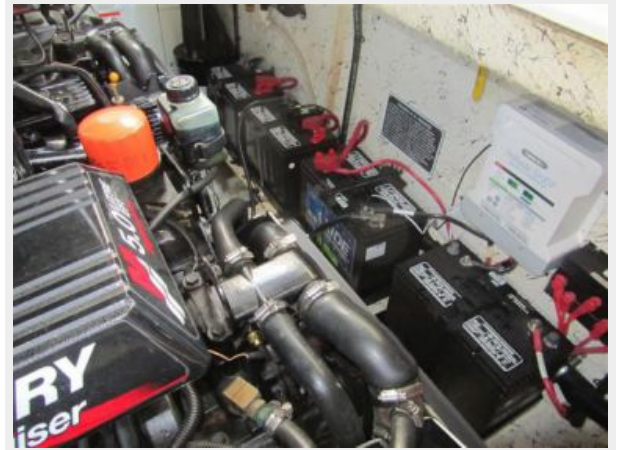
Rinker 310 Engine & house batteries
