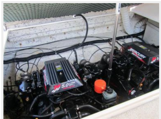
Rinker 310 Engine room
