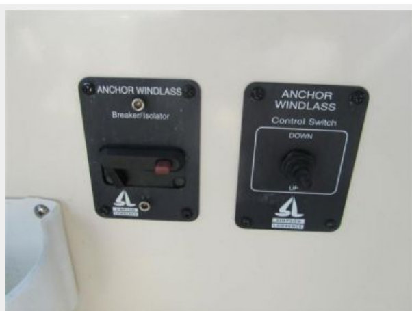
Rinker 310 Windlass breaker & helm controls
