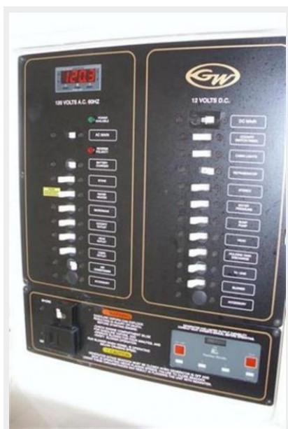
Grady White Electrical Panel
