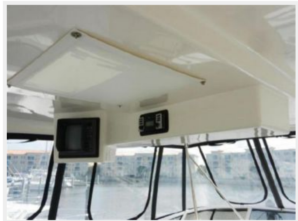
Bridge Overhead Electronics
