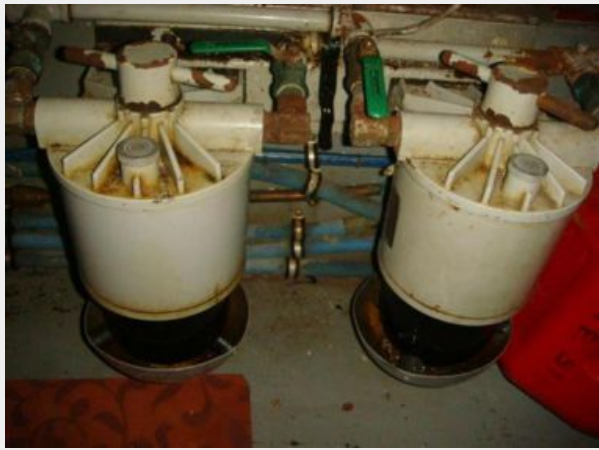
52' Hatteras Dahl fuel filters
