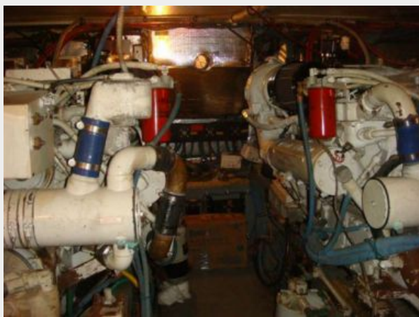
52' Hatteras engine room aft
