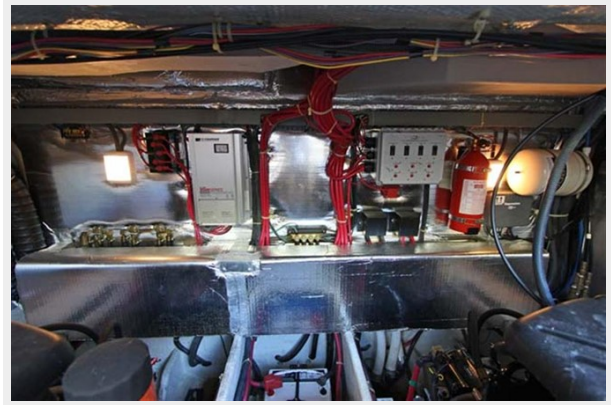
Engine Firewall W/Battery Charger, Main Breaker Panel, & Fire Suppression
