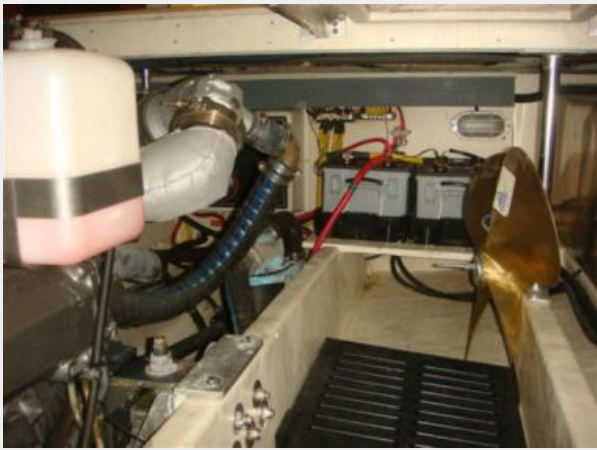
40' Mainship engine room aft
