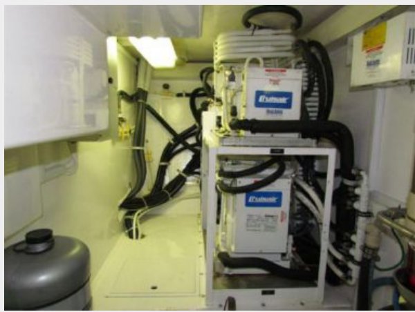
Machinery Rm Fwd w/Five Cruiseair Compressors
