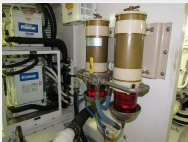
Dual Racor Fuel Filters
