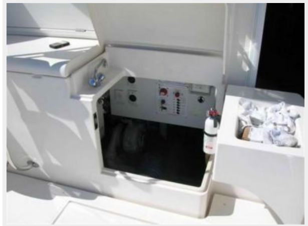
Engine Room Access
