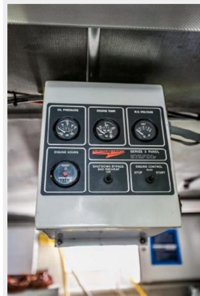
Engine Room - 30kw Northern Lights GenSet
