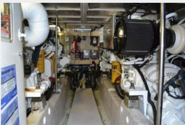
56' Sea Ray Engine room
