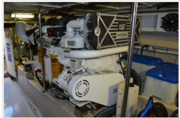
56' Sea Ray Engine room
