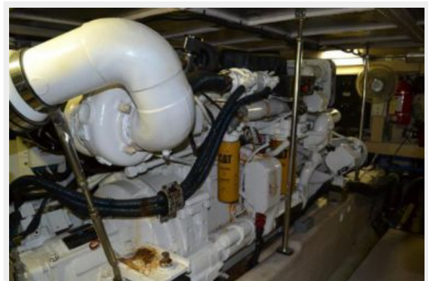
56' Sea Ray Engine room
