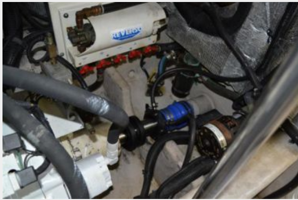
56' Sea Ray Engine room
