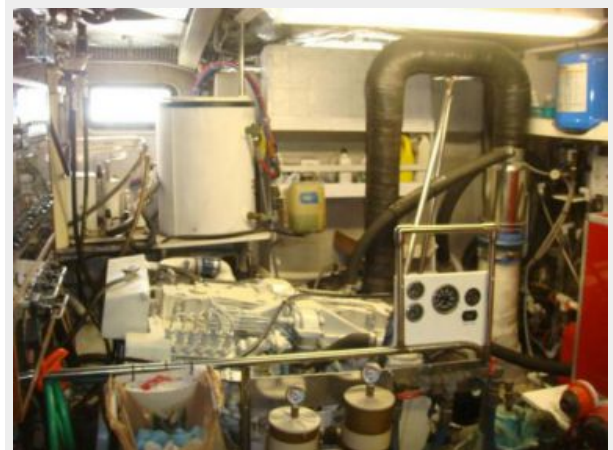
52' Cheoy Lee engine room starboard
