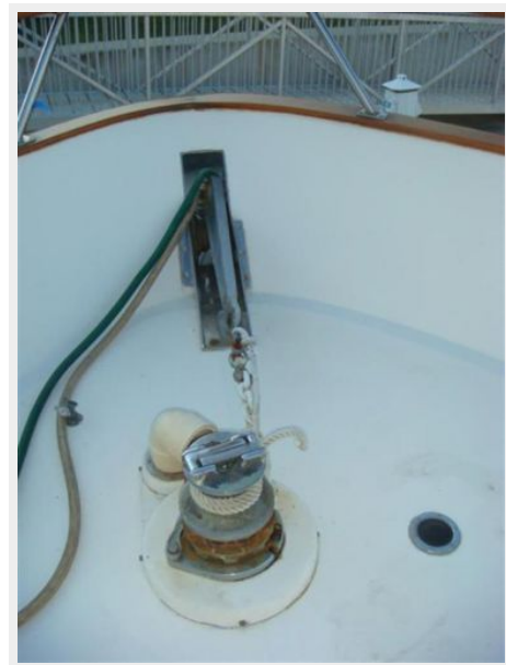
57' DeFever anchor windlass
