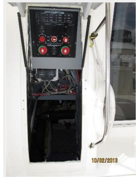
Engine Room Access
