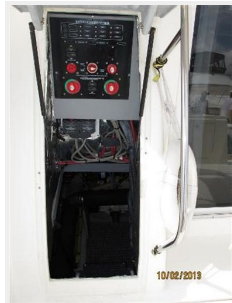
Engine Room Access
