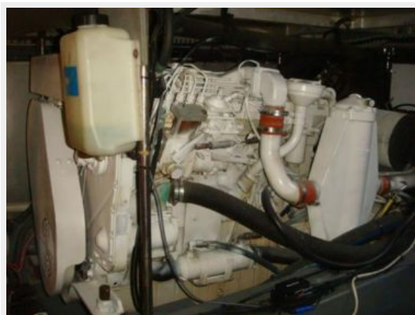
44' Carver starboard main engine photo1
