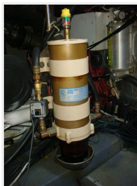
44' Carver starboard Racor fuel filter
