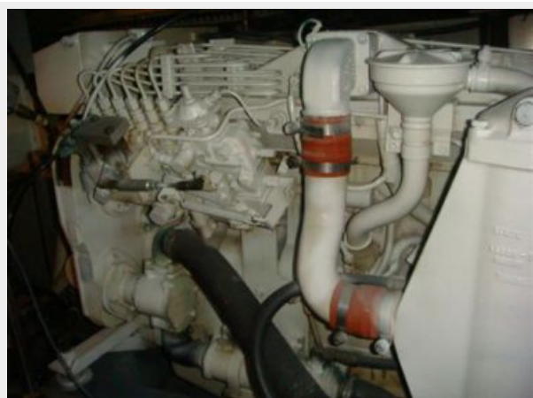
44' Carver starboard main engine photo2
