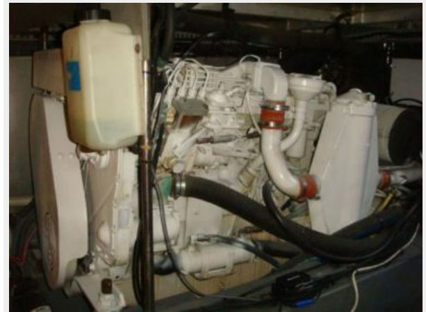
44' Carver starboard main engine photo1
