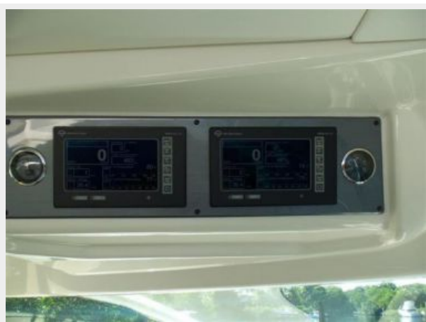
MAN Screens Overhead
