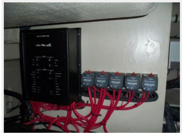
Electric Battery Switch
