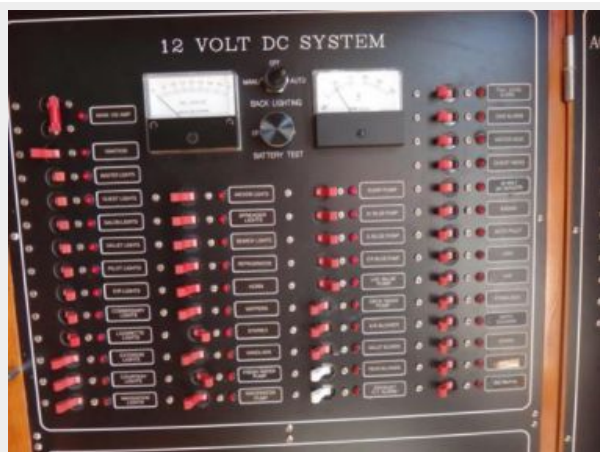
43' Selene electrical panel
