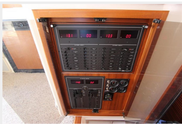
AC/DC Electrical Panel
