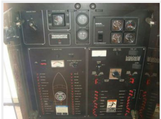
37' Bayliner electrical panel
