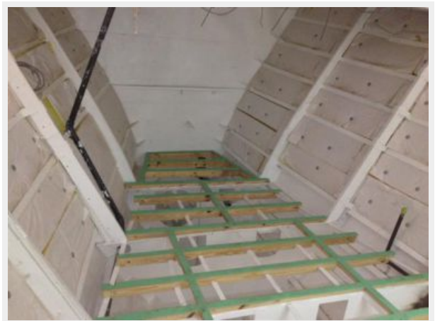
Floor Framing In Bow
